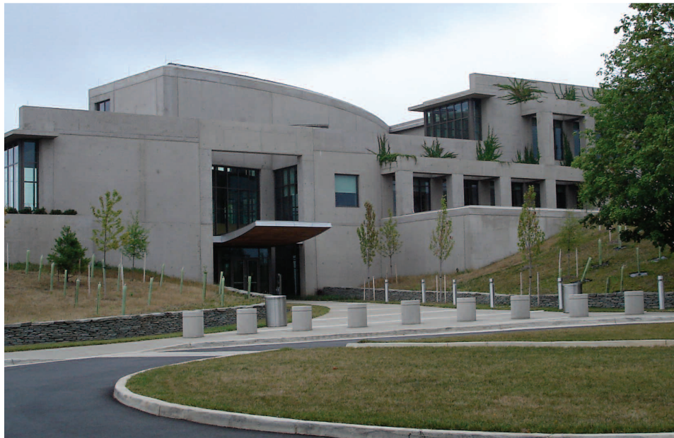
Linking Culpeper to Capitol Hill: Information Technology Services provides networking capabilities between the newly opened Packard Campus for Audio-Visual Conservation in Culpeper, Va., as seen in these two views, and the Library's reading rooms on Capitol Hill, approximately 60 miles away.
