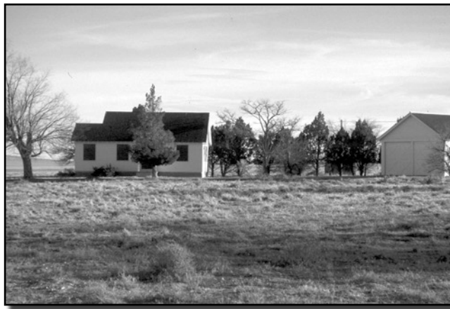
Buildings constructed in the 1930s at the Desert Range were typical Forest Service wood-frame structures.
