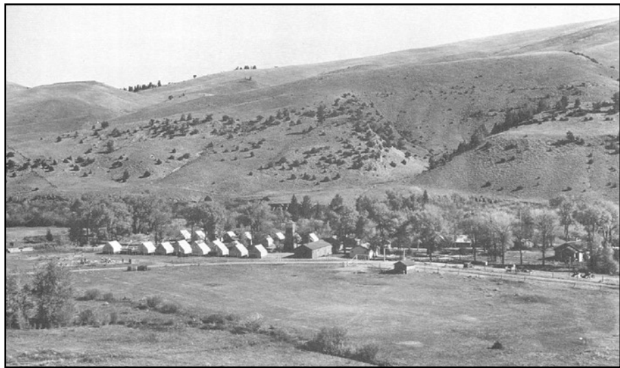
The first CCC camp in Region 1 was set up in 1933 at the Ruby River Ranger Station (Guth and Cohen 1991) where the Vigilante Experimental Range was established in 1935. The building at far right, erected before 1925, became an experimental range cottage.
