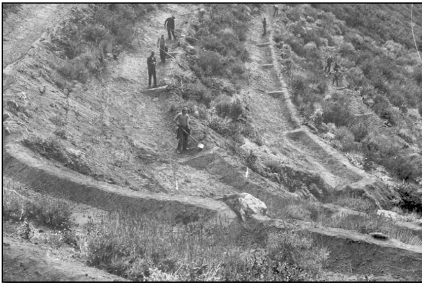
Contour trenches were constructed (above) by CCC workers at the head of Ford Canyon in Davis County in 1934. The same area (below) as it appeared in 1945.
