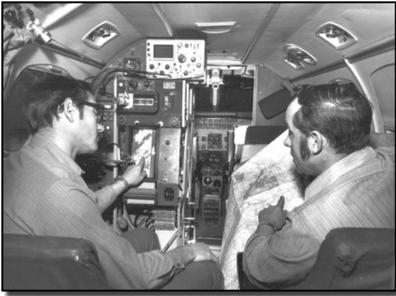
Electronic Technicians John Voth (left) and Dale Gable used an infrared sensor inside an aircraft in 1971 to locate small forest fires, record the imagery, and identify a ground location with the interpreter's map.
