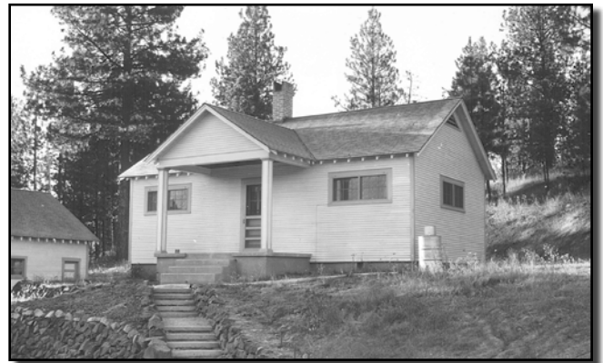
A dormitory building constructed in 1933 on what was known as "Research Hill" at the Boise Basin Branch Station at Idaho City.
