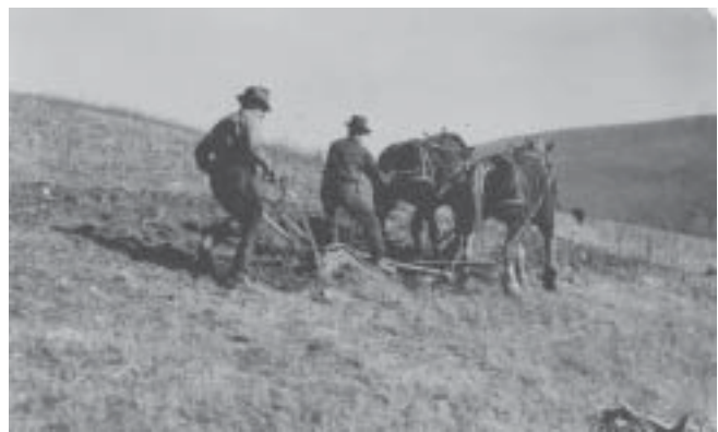
Figure 80 —Wasatch Plateau: building contour trenches with horse and plow during the 1920s.
