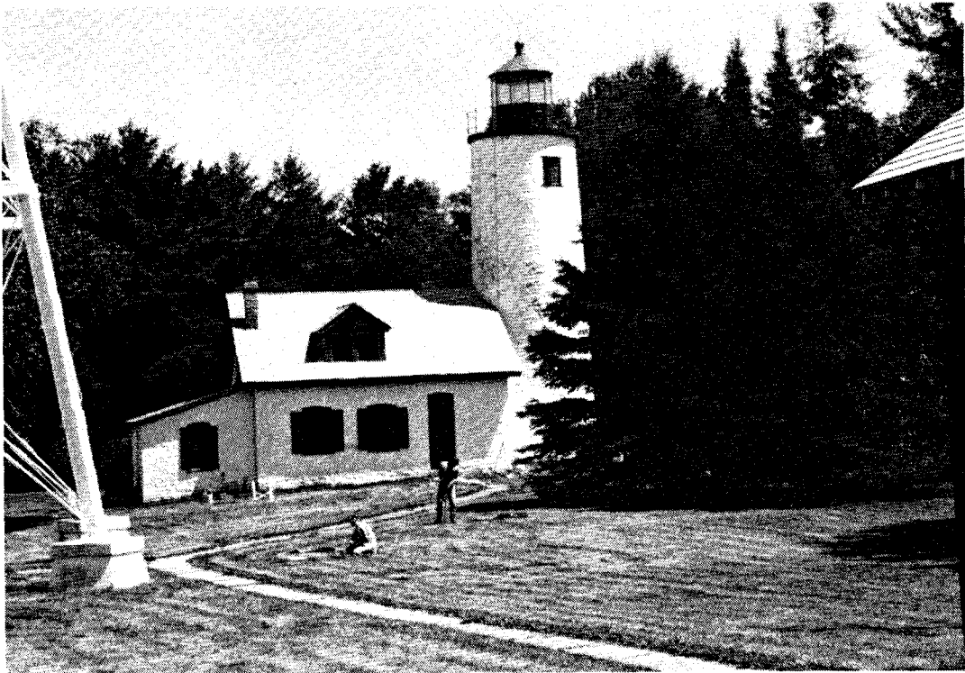
Figure 12. Old Michigan Island lighthouse, 1988.
