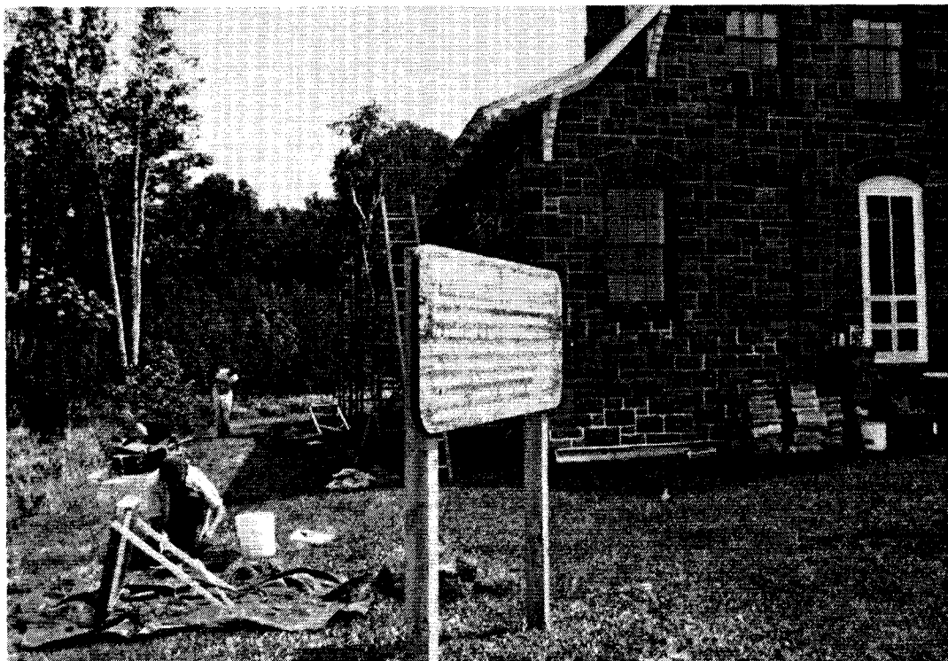
Figure 7. Sand Island complex, 1988.
