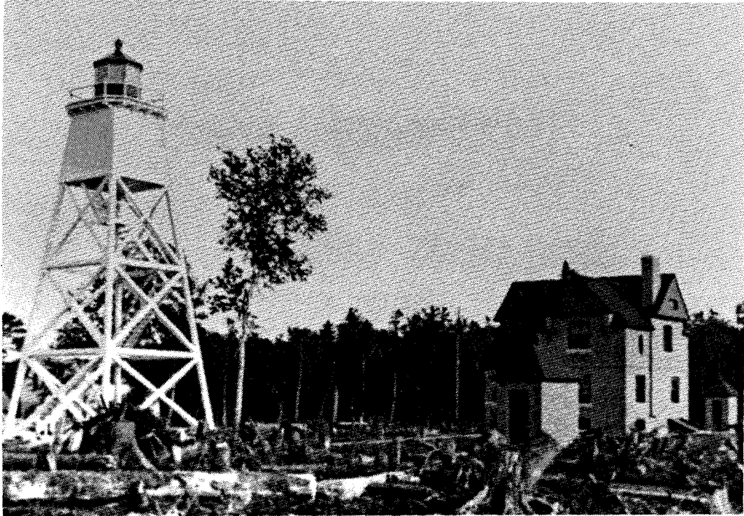
Figure 30. Devils Island east keeper's quarters and original tower shortly after construction.
