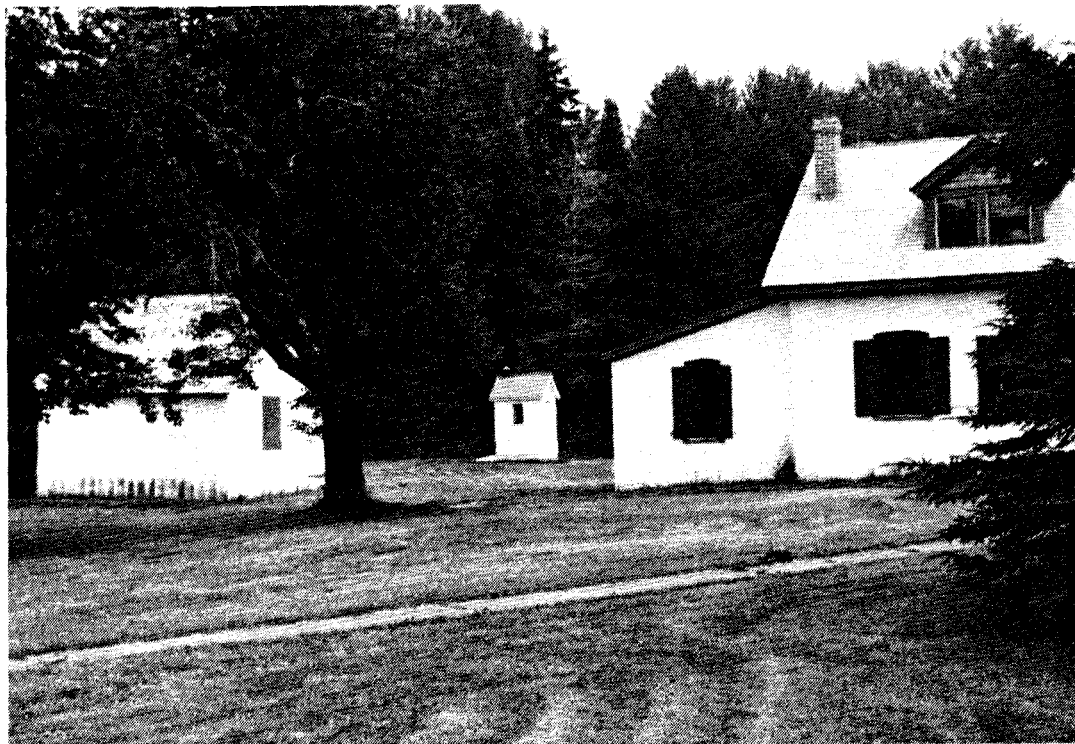
Figure 17. Michigan Island old lighthouse shed addition and outbuildings, 1988.
