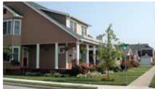
Affordable homes at Cowart Place, a mixed-income development built in downtown Chattanooga by CNE
