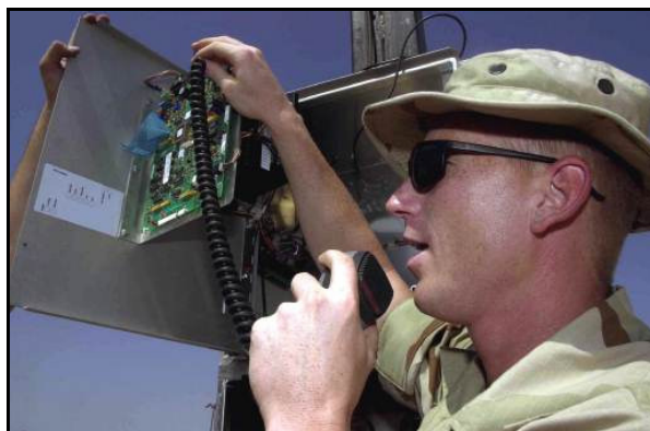
Figure 4.27. Mass Notification System.
