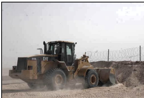
Figure 2.1. Berm Construction.
