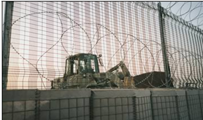
Figure 4.23. Obscuration Screen on Perimeter Fence.
