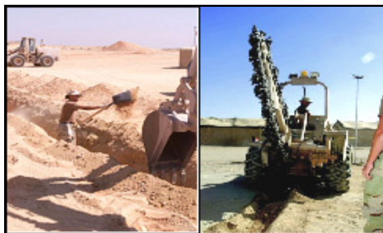
Figure 4.37. Burying Utility Lines.
