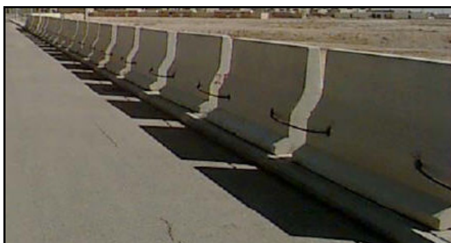
Figure 4.19. Jersey Barriers Cabled Together.
