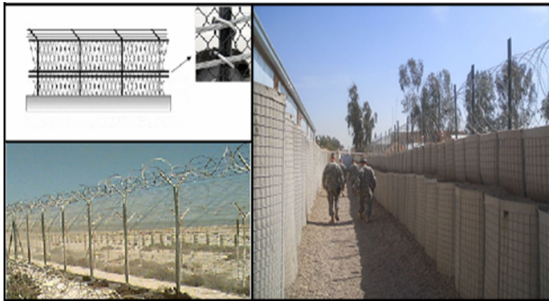
Figure 4.15. Perimeter Fences and Barriers.
