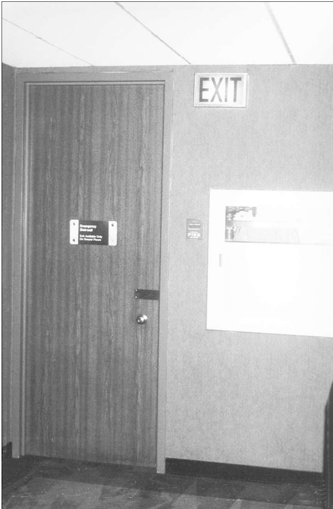
10. Typical exit arrangement at rear of floor, South Tower.
