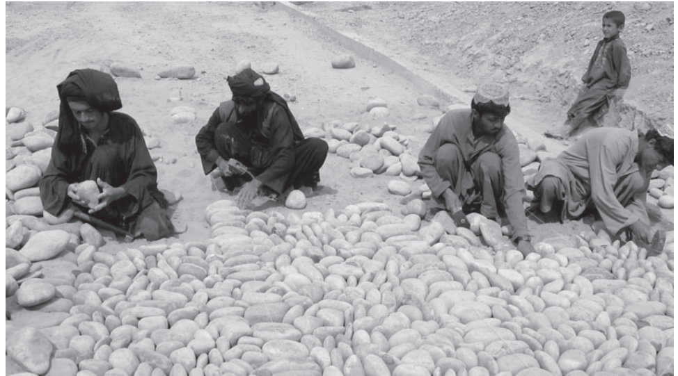
Figure 4: Cash-for-Work Road-Construction Project
