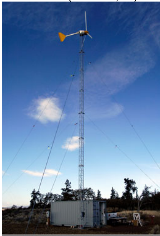
Photo 2: Turbine installed on Kennell property Source: NWSEED
