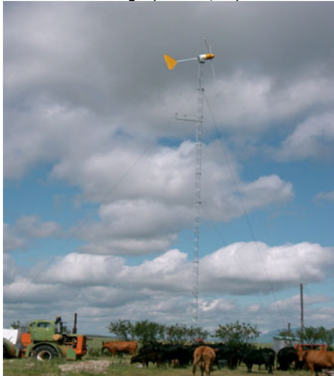
Photo 1: Turbine installed at Alger ranch Source: NWSEED
