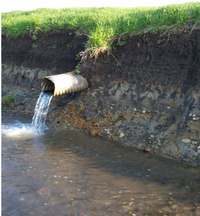
Figure 10. —A 10-inch main tile outlet into a surface drainage ditch in an area of Drummer and El Paso silty clay loams, 0 to 2 percent slopes.
