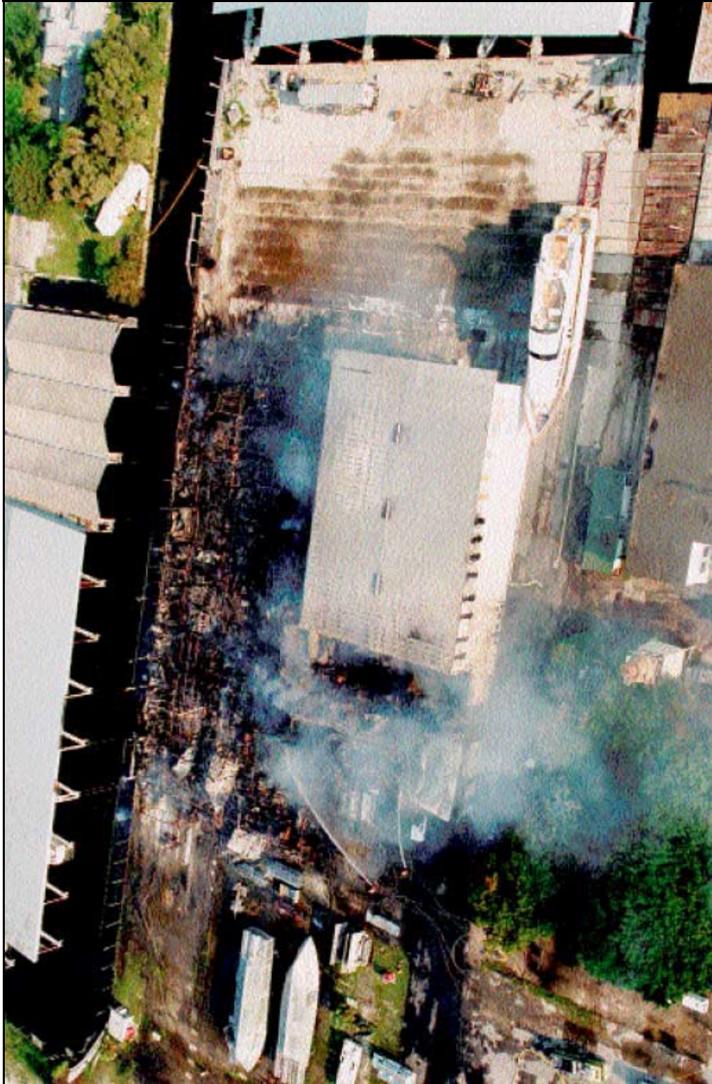
5. Aerial view of the fire scene, with the canal and neighboring covered boat slips (to the west) at top of photograph.
