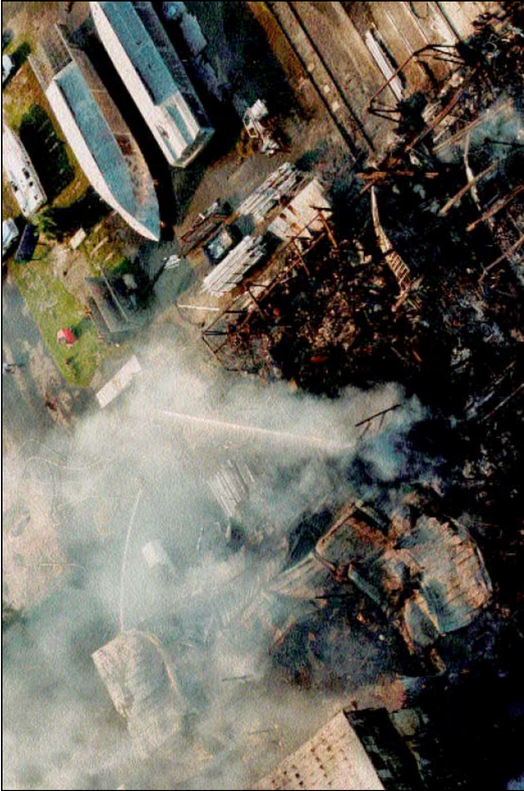
4. Aerial view of the south corner of the collapsed Manufacturing Building (Building A).
