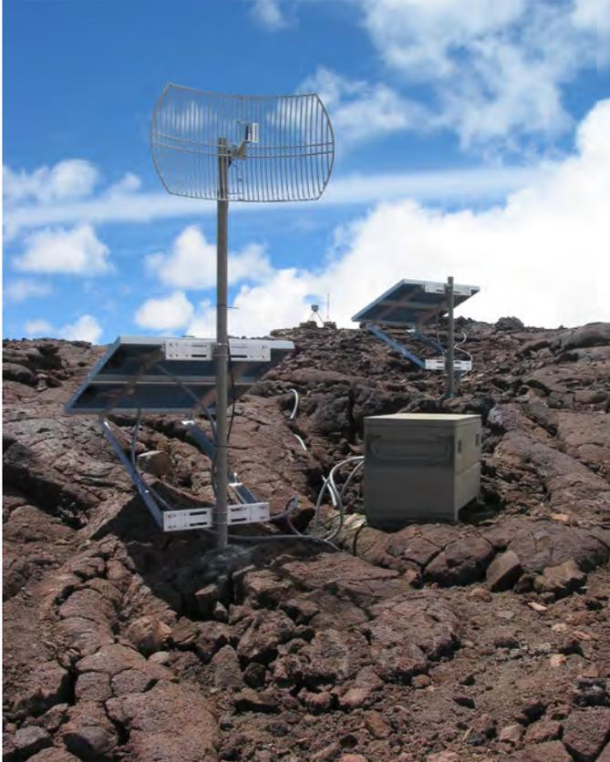
**Figure 12.** Hyperlink Technologies model HG2424G antenna at the camera node on Mauna Loa. The pipe supporting the antenna also supports two 60 watt solar panels; the other pipe supports two additional 60 watt panels. The radio, four charge controllers, and eight batteries are in the steel box. The camera enclosure, which is on the caldera rim, is visible in the background.
