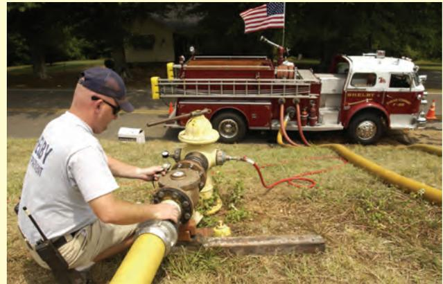
A Shelby firefighter checks a setup whereby a fire truck is used as a pumping station to pump 870 gallons of water per minute from the Shelby municipal water supply through a fire hydrant connected to the Cleveland County water system to a Kings Mountain pumping station 8,000 feet away.
