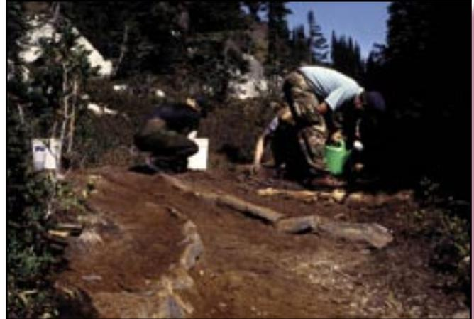
Figure 1–5b— This trail at Lake Mary was narrowed using rocks so the margins could be restored.
