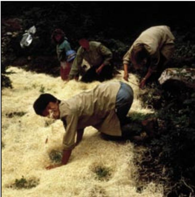
Figure 3–134—When it’s time to roll out the carpet (the erosion-control blanket in this case), there is a great sense of satisfaction, nigh unto gaiety. The hard work to prepare and plant a site is almost done!
