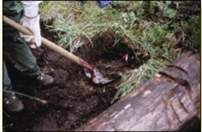
Figure 3–53b—In gullies, a keyway is excavated about 6 inches into each sidewall to pin the checkdam or siltbar material into place.
