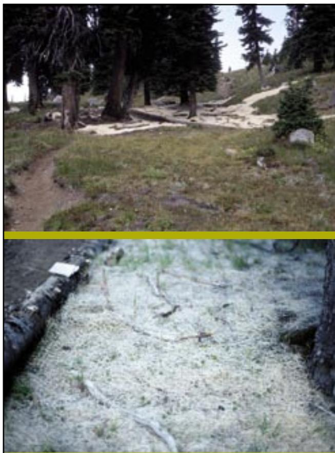
Figure 3–138a and 138b—Erosion-control blankets made of excelsior (aspen shavings) are alarmingly bright when they are first rolled out (top). After 1 year, they begin turning gray (bottom).
