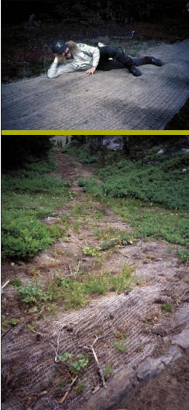
Figures 3–139a and 139b—Coconut Man sports a wig showing off the dark brown color of a freshly unfurled coconut fiber erosion-control blanket (top). At this subalpine site, the coconut matting had begun deteriorating (bottom) 4 years later.
