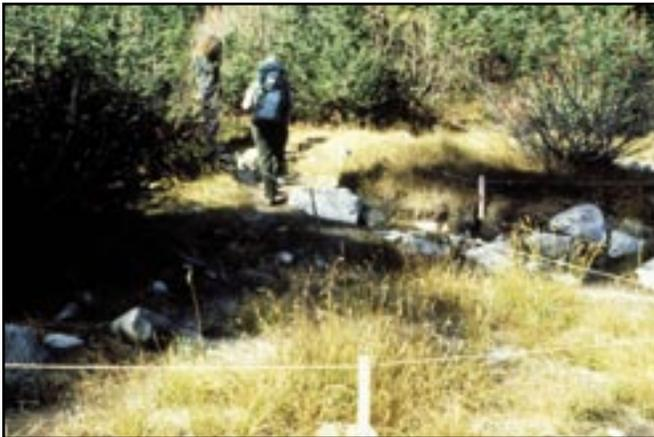
Figure 3–85a—While string fences can rope off large expanses or block a trail, they require perpetual maintenance.
