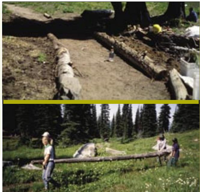
Figure 3–82a and 82b—These low-profile log barriers (top) delineate a trail through a closed restoration site. The barriers also serve as silt dams for backfilling the restoration sites. Log carriers (bottom) placed underneath the log are useful when transporting log barriers.
