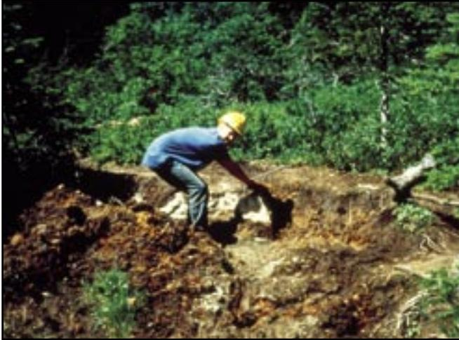
Figure 1-10—A deeply incised trail at Lake Valhalla in the Henry M. Jackson Wilderness, WA. Once an erosion channel forms, water—rather than foot traffic—causes most of the damage.
