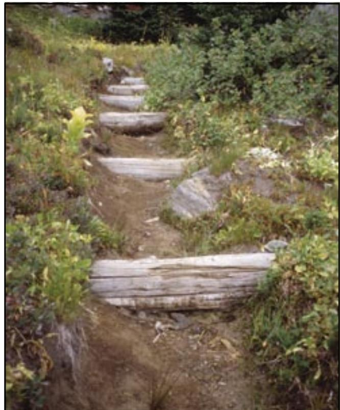
Figure 3–50—Log checkdams are an example of a nonliving subsurface erosion control structure. The checkdams are keyed into the bottom and sides of an eroded hiking trail, preventing further erosion and collecting sediment.
