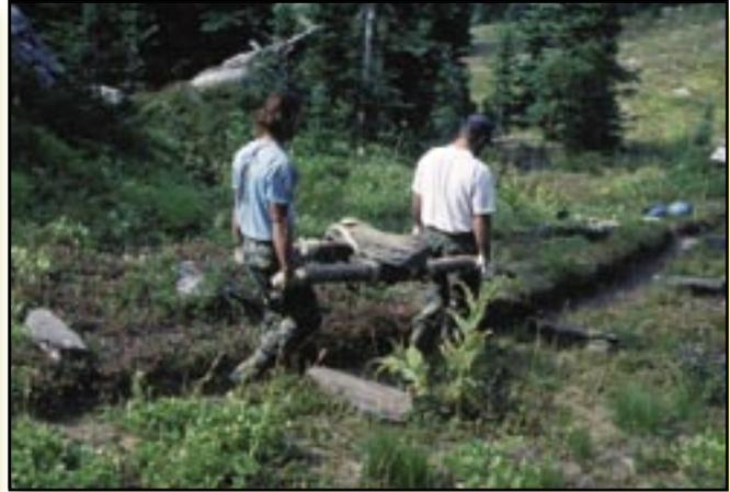
Figure 3–78—Litters can be improvised to move rock. Grip hoists can be used to drag larger rocks, but doing so would damage vegetation.
