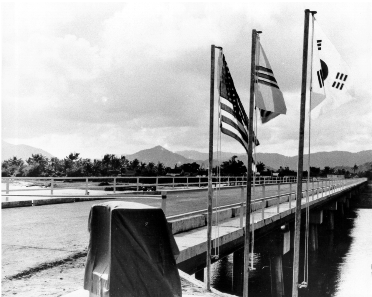
The completed Ban Thach bridge was dedicated on 7 December 1968.
