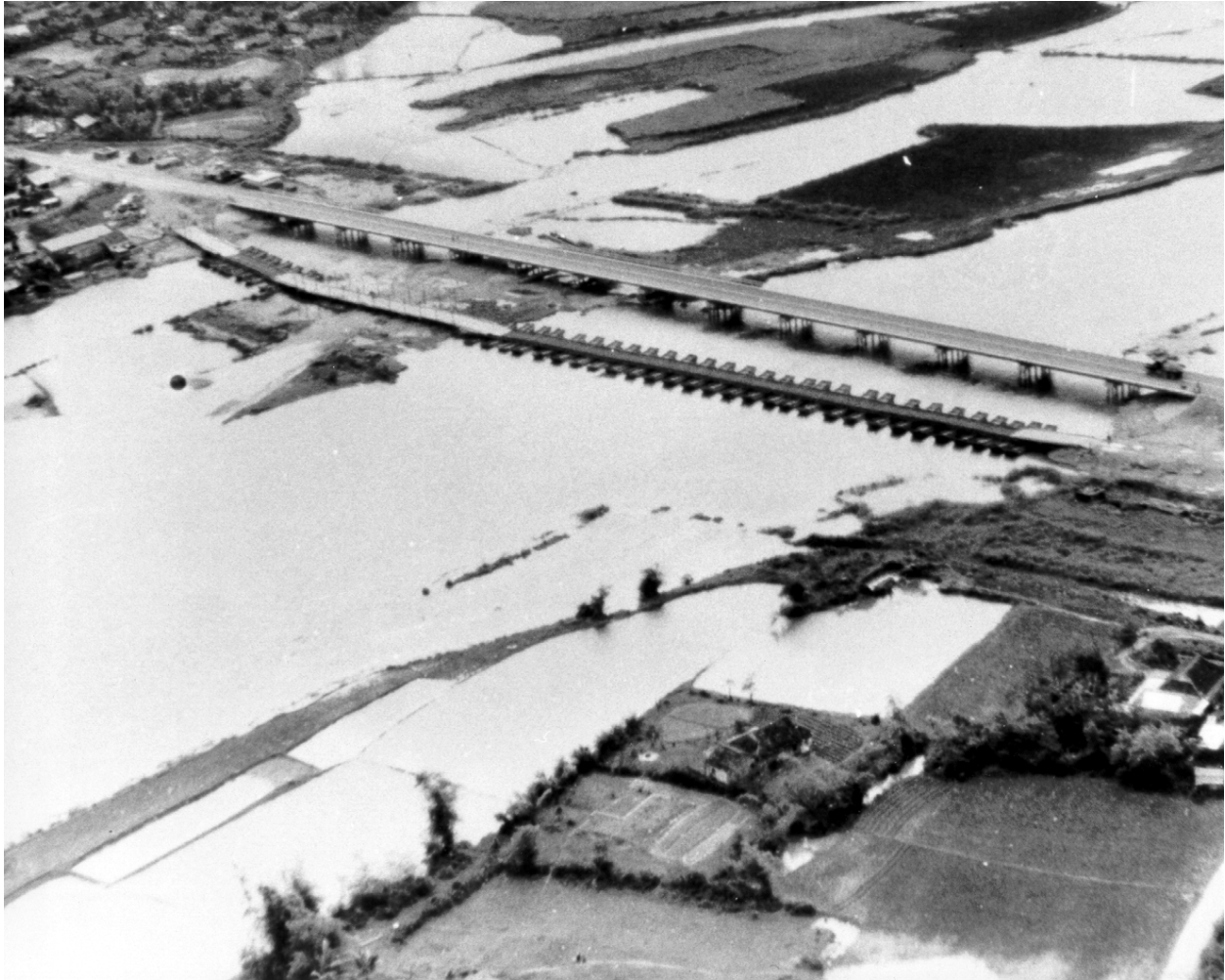
Army Engineer bridges over the Ban Thach River in South Vietnam. In the foreground was an M4T6 bridge and the background an 840-foot, 13-pier bridge.
