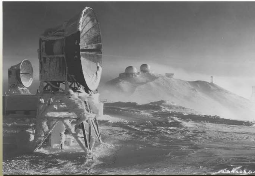
DEW Line radar stations located in Alaska
