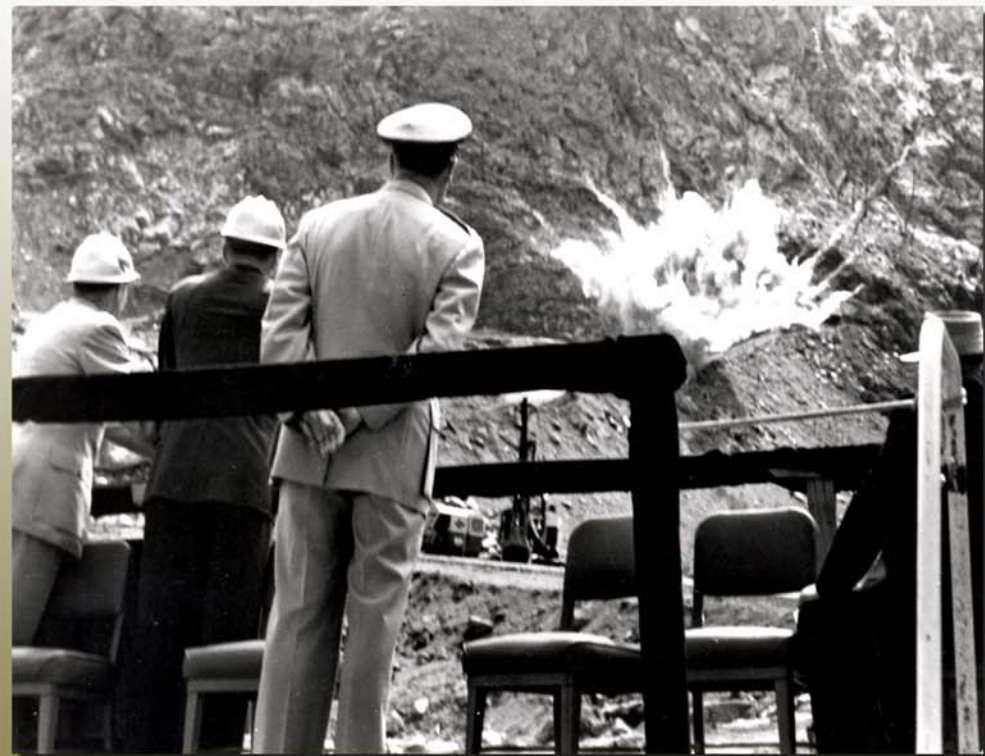
16 June 61: First blast to begin construction at Cheyenne Mountain Complex
