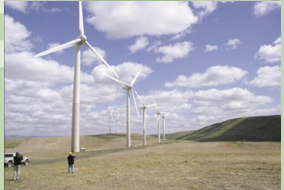
Combine Hills Wind Project, Milton-Freewater, Oregon
