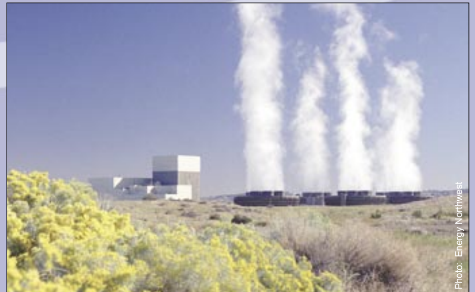
Columbia Generating Station, Richland, Washington
