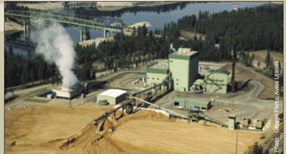
Kettle Falls Generating Station, Kettle Falls, Washington
