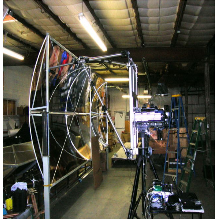
Figure 8. The VSHOT test setup at Industrial Solar Technology's facility in Golden, Colorado.
