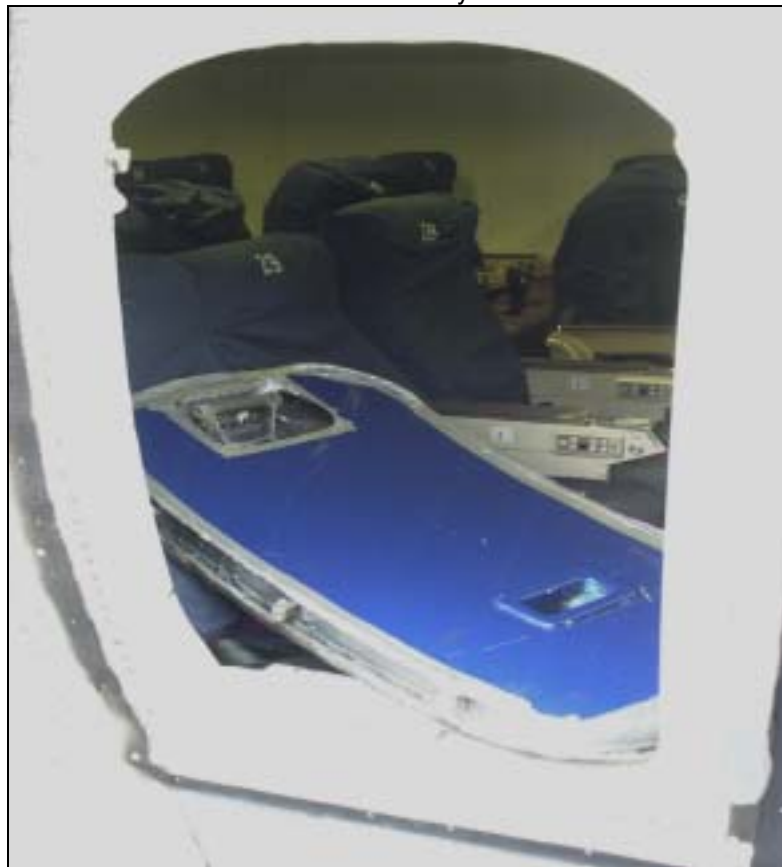
Figure 29 Exit Obstructed by Hatch
