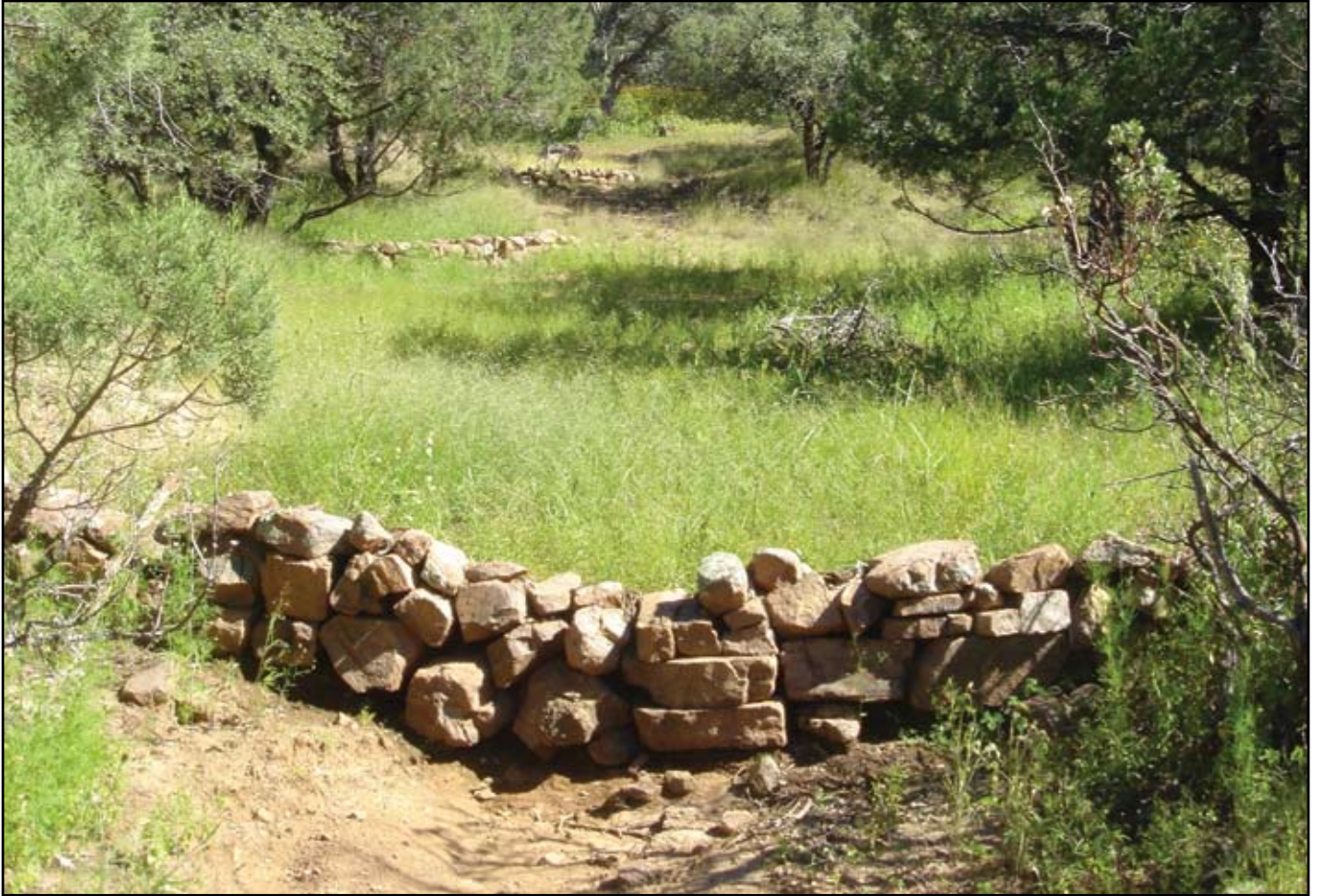
Loose rock structures successfully collecting soil and generating vegetation growth.
