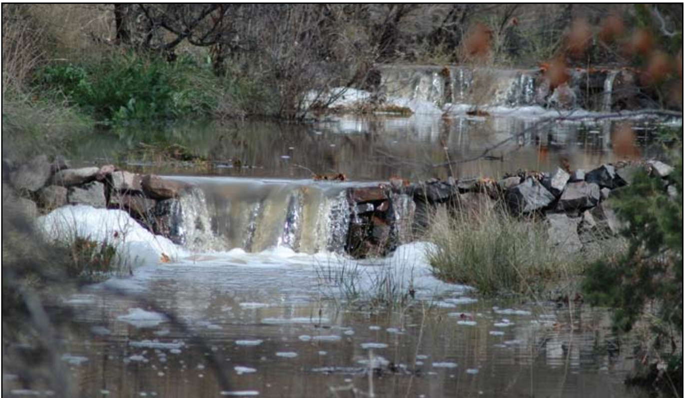
Loose rock structures withstanding flood waters.
