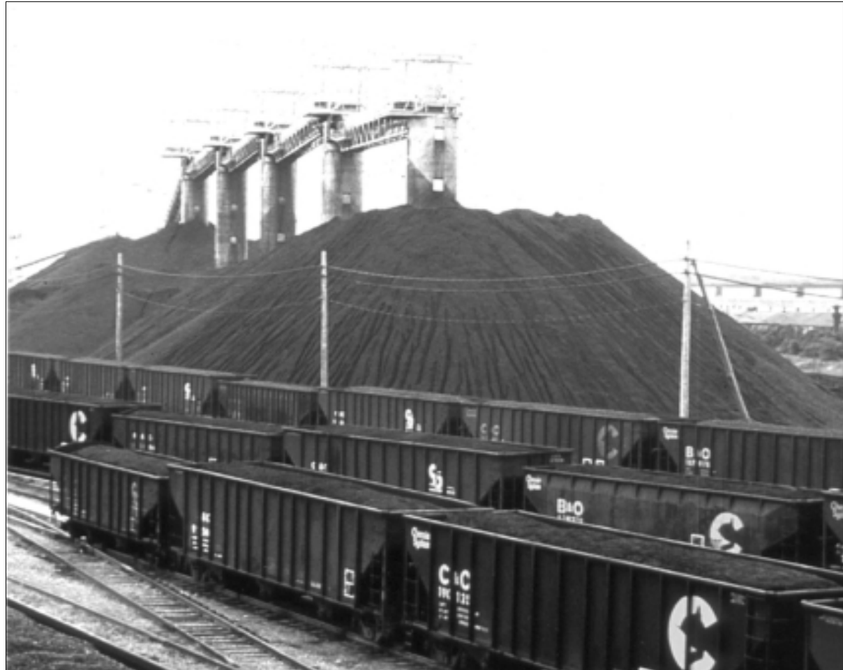
Coal yard, Curtis Bay, Maryland. Source: U.S. Department of Energy.
