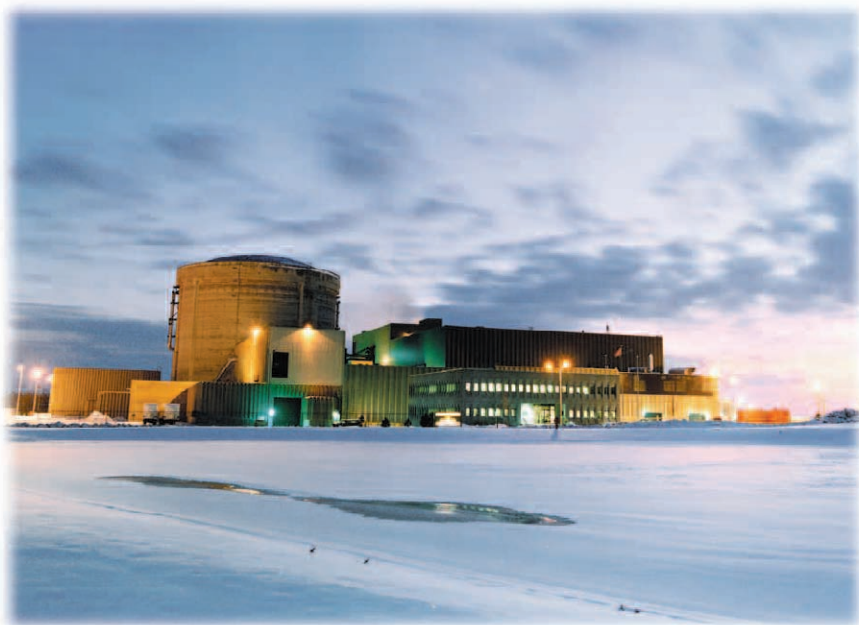
Point Lepreau CANDU 6 Nuclear Generating Station.
