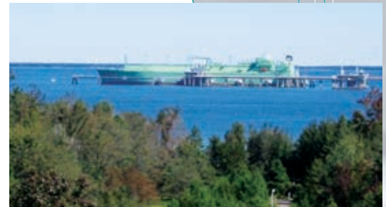
LNG is pumped from ship to insulated storage tanks
