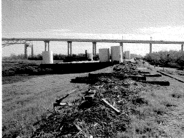
Figure 4.17: Debris line near levee crest just west of the Rt. 47 Bridge south abutment (L. Wooten, October 5, 2005).
