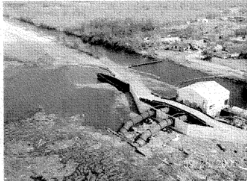
Figure 5.3: Aerial photograph of levee breach of hurricane (back) levee at levee transition near Hayes Pump Station (September 25, 2005)
