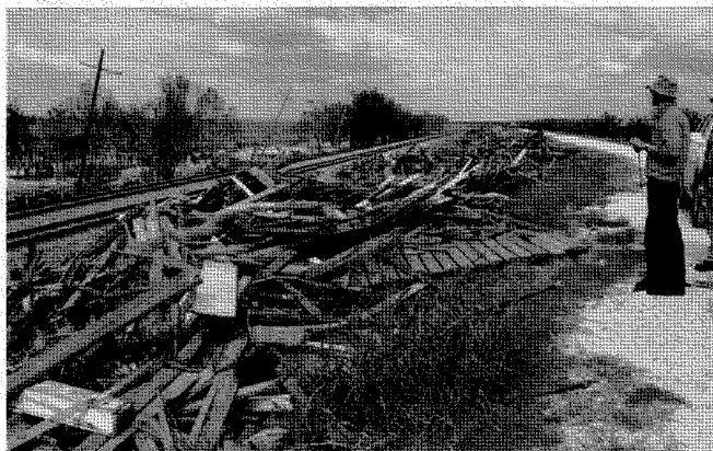
Figure 3.8: Debris from the Little Woods houses accumulated near the crest of the earth levee indicates the level of the lake waters during the storm. (N 30° 04' 70.5", W 89° 56' 44.0")
