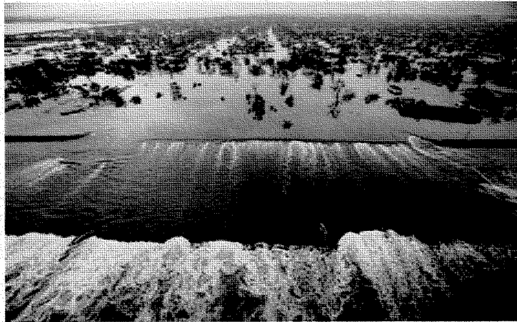
Figure 1.7: Flooding at the west end of the Ninth Ward, and outflow through levee breach as initial storm surge subsides.
