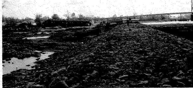
Figure 4.6: South view of the south breach repair at the Lower Ninth Ward (J. Wartman, October 4, 2005).
