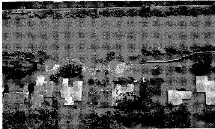
Figure 2.15: The breach section at the west side of the London Avenue Canal (North).
