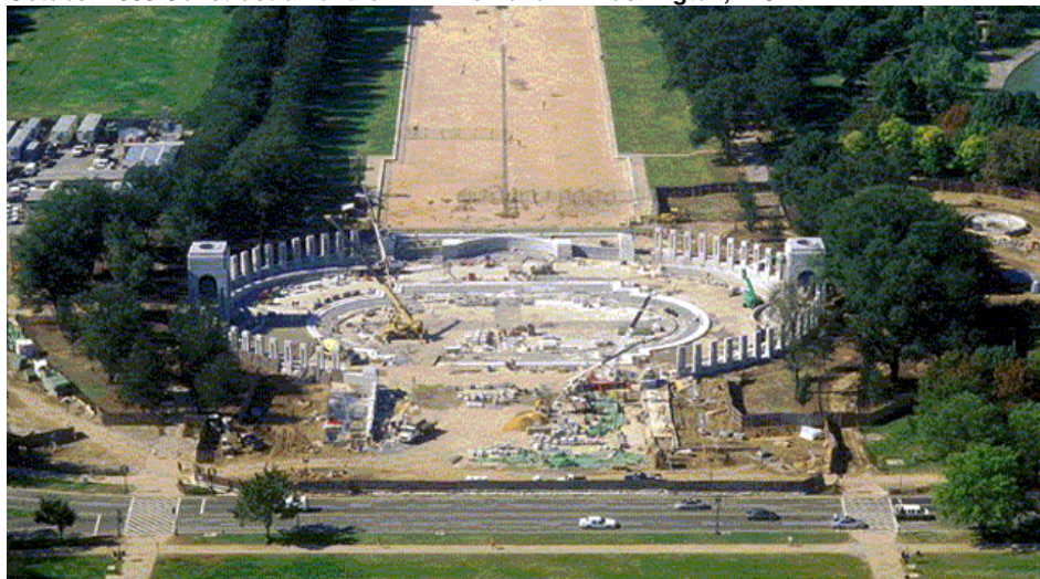
October 2003 Construction of the WWII Memorial in Washington, D.C.
