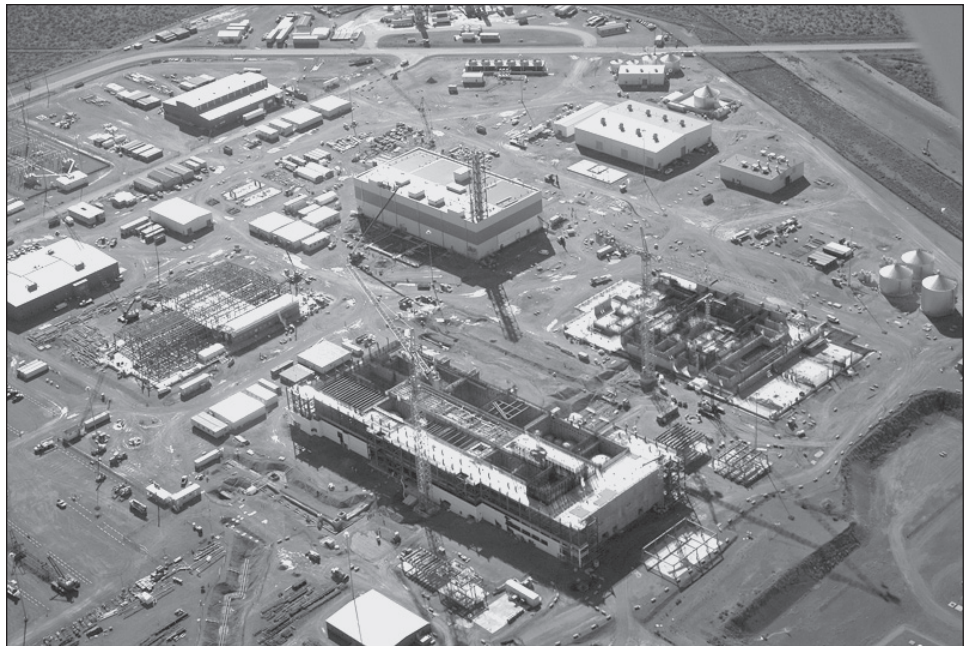
Figure 1: Aerial View of Hanford Waste Treatment Plant under Construction
