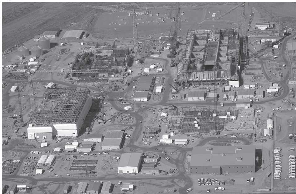
Figure 7: Aerial View of the Waste Treatment Plant under Construction at Hanford
