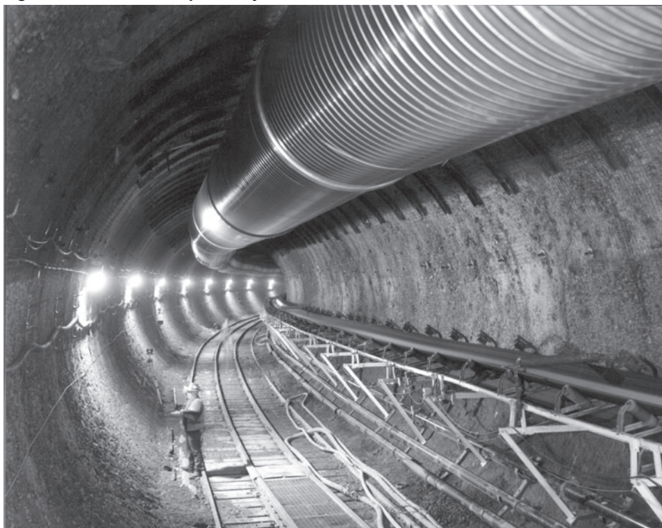
Figure 9: View of an Exploratory Tunnel at Yucca Mountain
