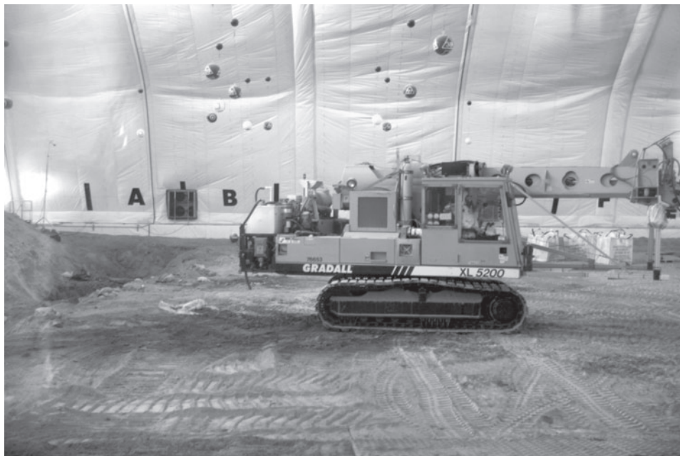
Figure 10: An Excavator Removes Buried Transuranic Waste at Energy's Idaho Cleanup Location
