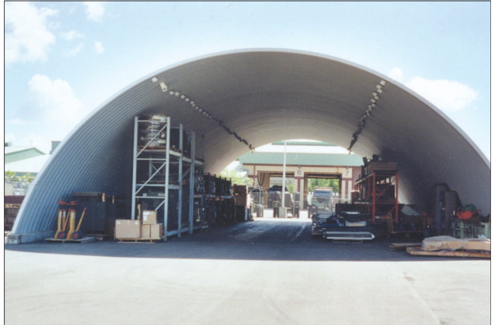
Figure 8: K-Span Shelter at Army Reserve Unit Fort Shafter, Hawaii
