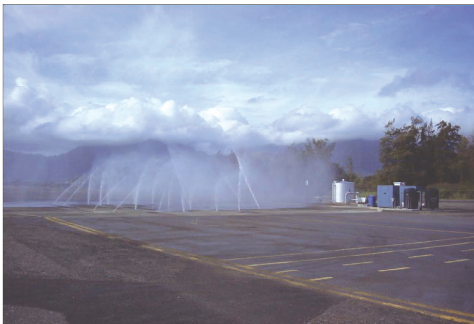
Figure 6: Marine Corps Helicopter Rinsing Facility Kaneohe Bay, Hawaii
