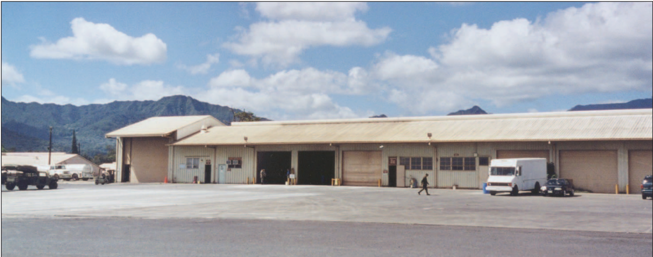
Figure 10: Corrosion Inhibitor Application Facility at Army's Schofield Barracks, Hawaii
