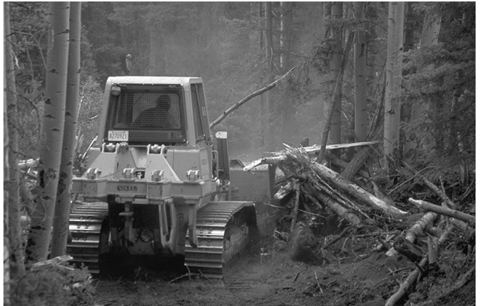
Figure 7: Bulldozer Piling Thinned Trees (Machine Piling)
