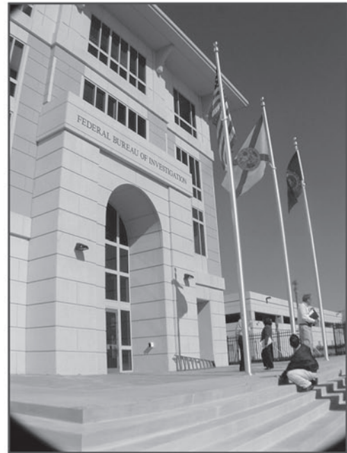
FBI Field Office, Tampa, Florida
