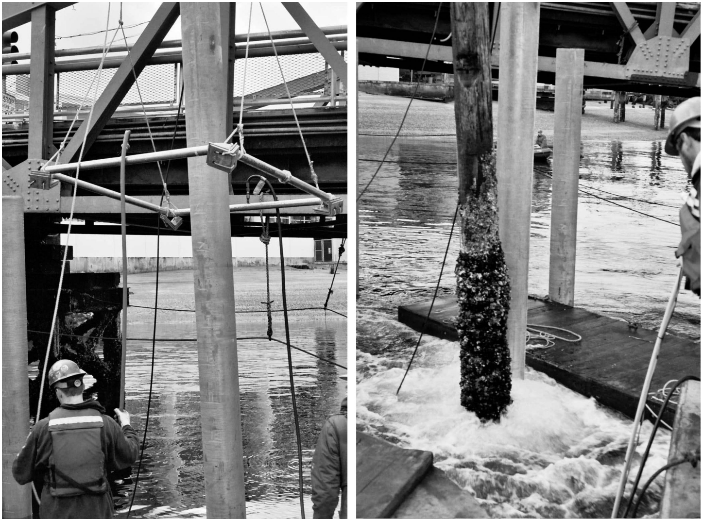
Figure 16: Replacement of Creosote-Treated Wood Pilings with Steel Pilings
