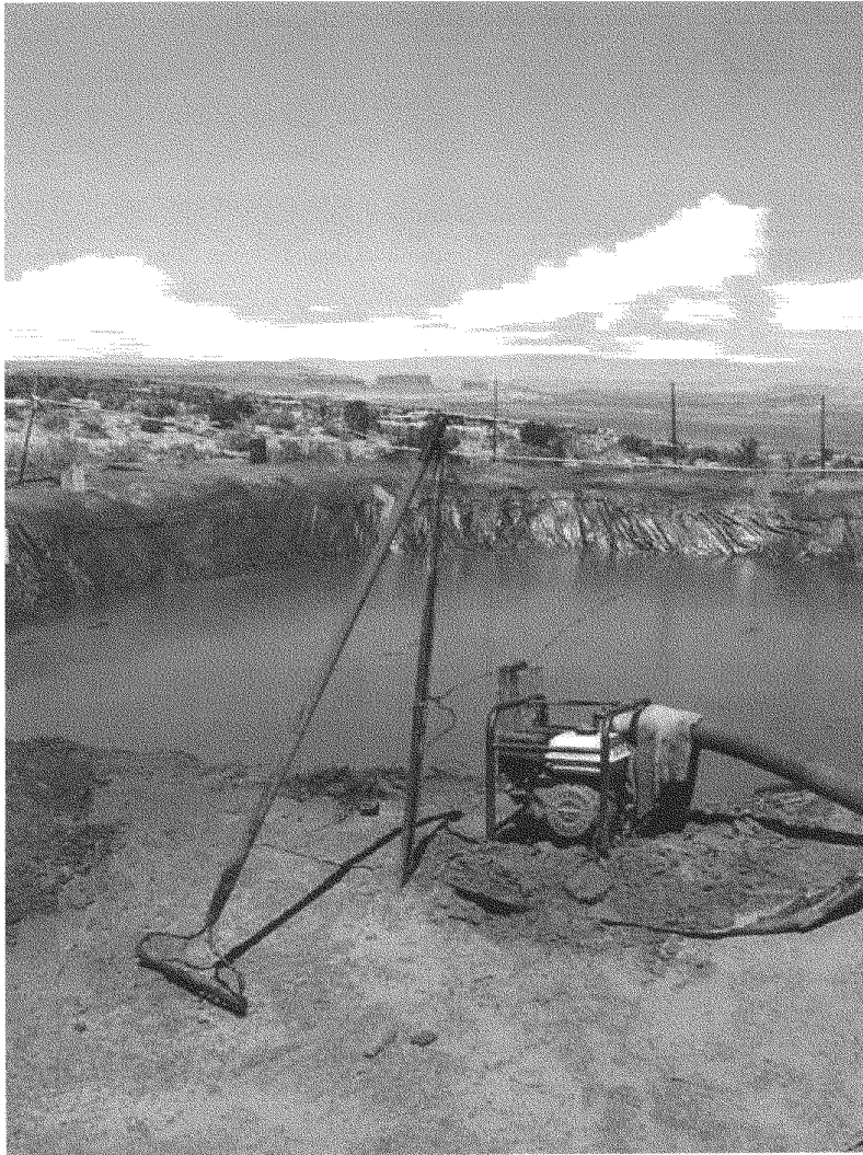
Sludge Pit at Long Canyon Well Outside Moab, Utah
