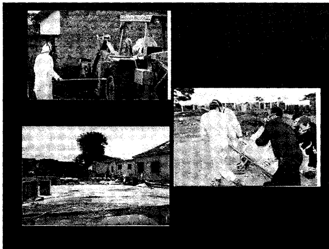
Photos of the scrap yard, demolition of a building and carting of contaminated soil.
