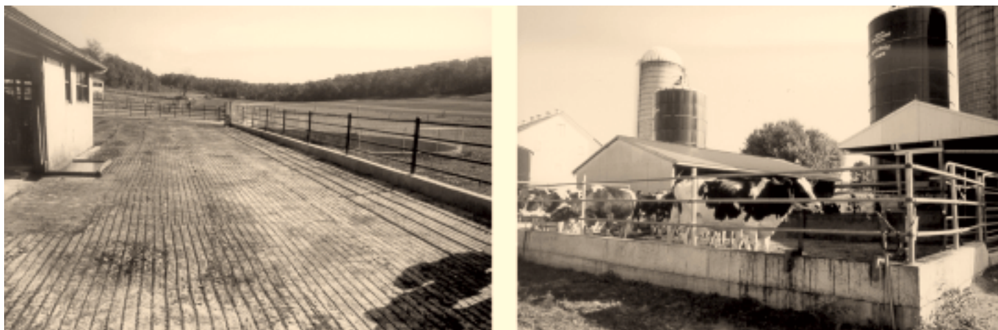
Figure 1: Cemented and Curbed Barnyards
