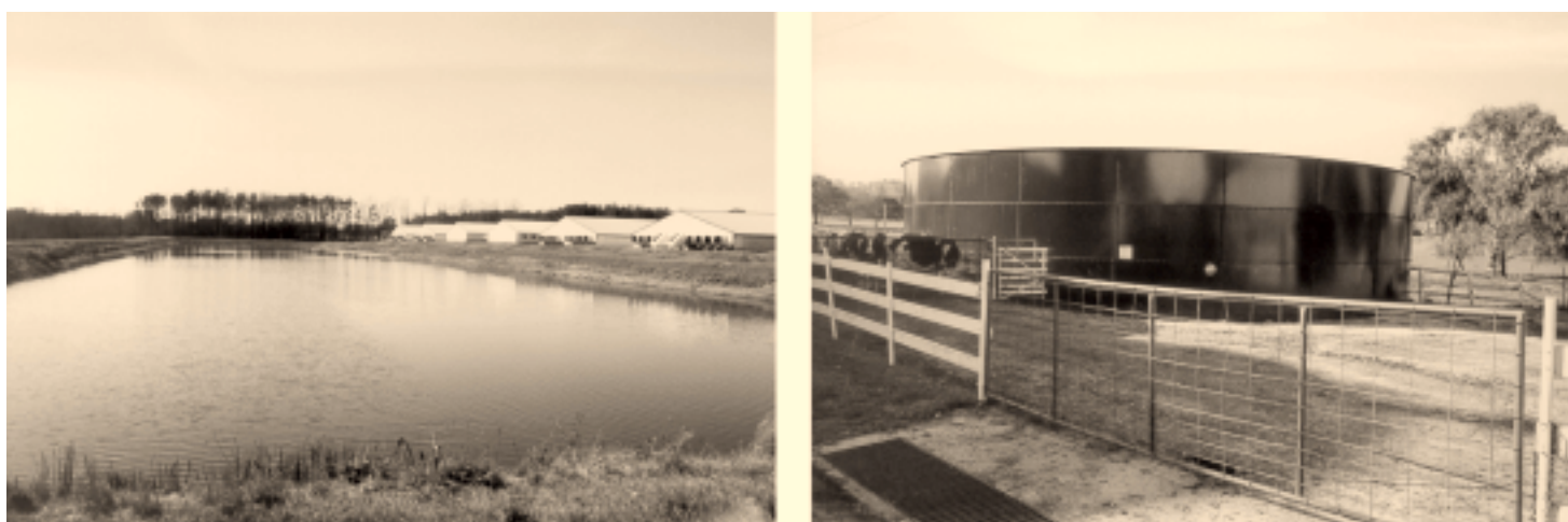
Figure 4: Storage Lagoon for Hog Waste and Storage Tank for Dairy Cow Waste
