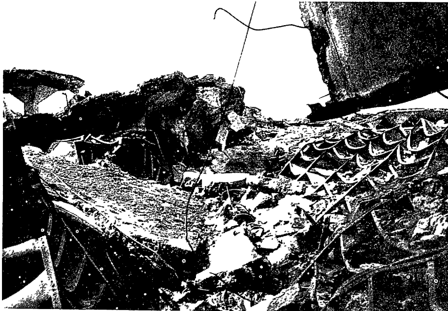
VIEW OF BUILDING CRUSHED BY COLLAPSED ROOF AFTER ST. LOUIS FIRE (Courtesy of General Services Administration)
