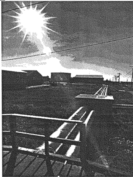
(RIGHT) PIPED WATER AND SEWER SYSTEMS: Permafrost (permanently frozen soil) prevents water and sewer utilities from being buried in many northern Alaskan communities.
