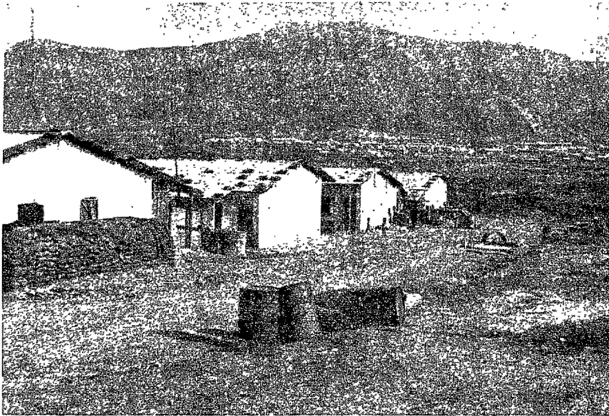
Shelters constructed near Da Nang, Military Region 1, for dependents of Vietnamese Army personnel
