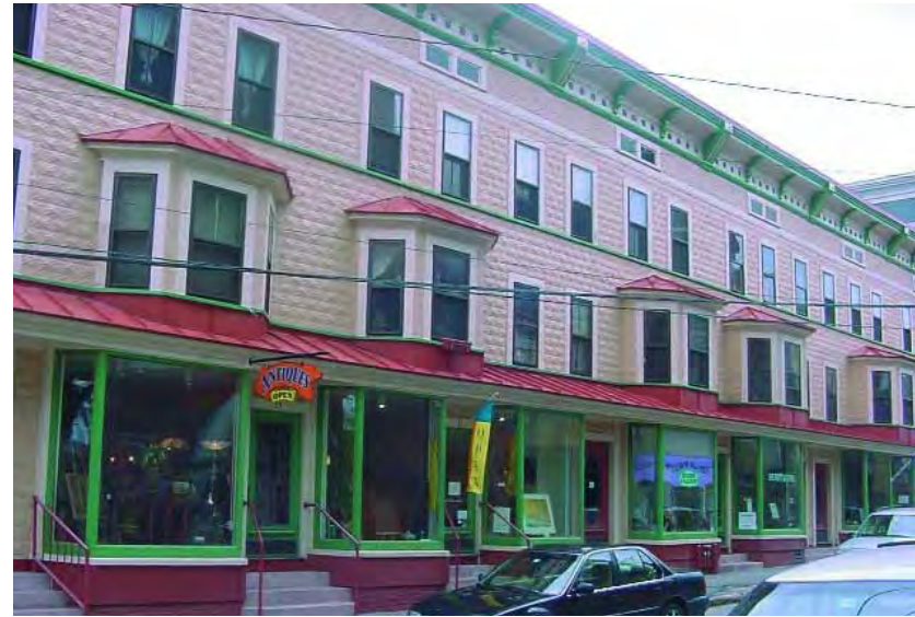
The Exner Block, Bellows Falls, courtesy of the Rockingham Arts and Museum Project.
