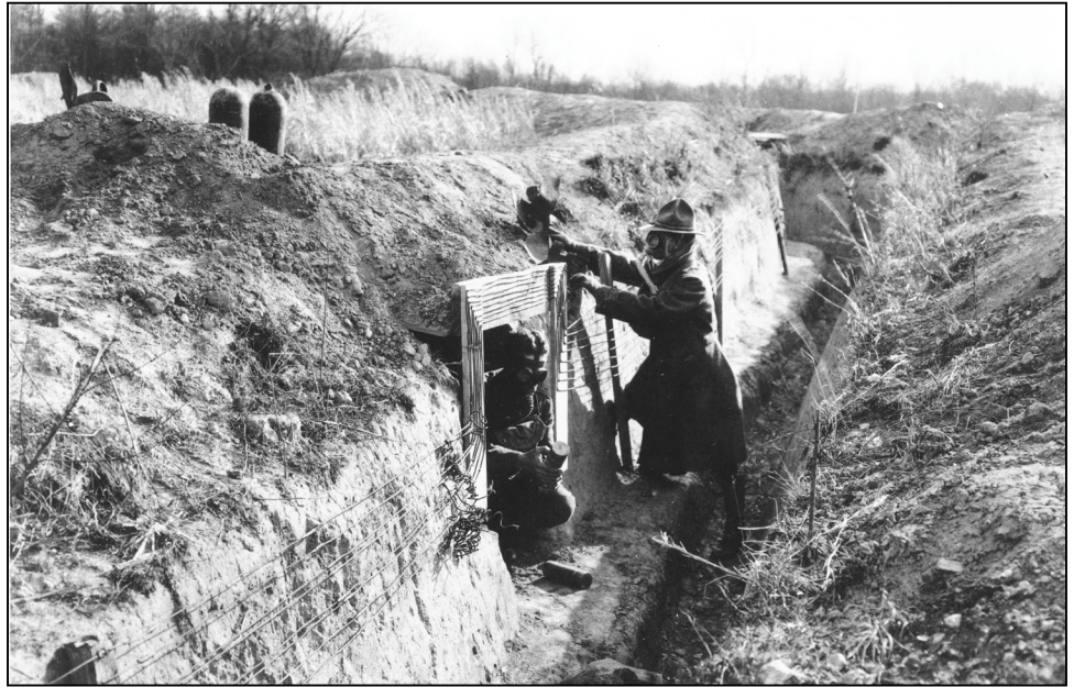
Figure 1: World War I-era Photograph of Two Soldiers Preparing to Test Chemical Munitions in a Trench Located in Spring Valley
