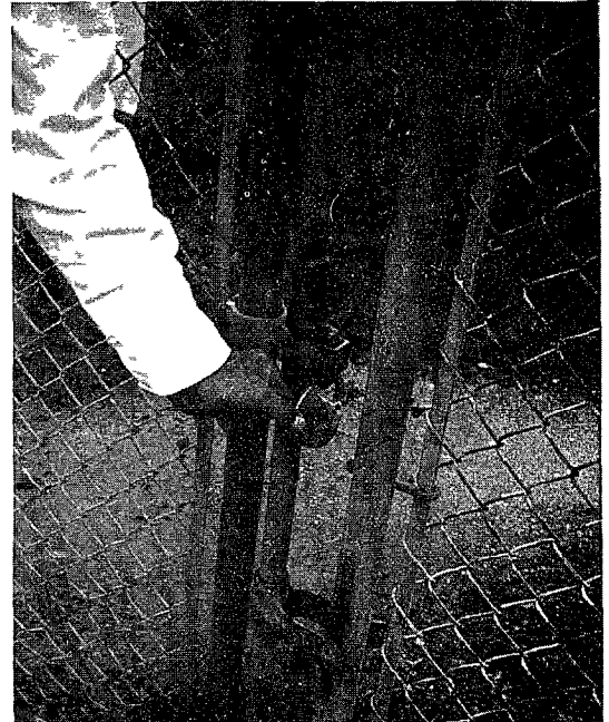
Lock opened when pulled
