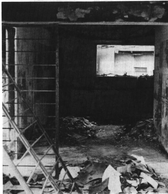
Damage to an embassy officer's home during the FMLN offensive in San Salvador.
