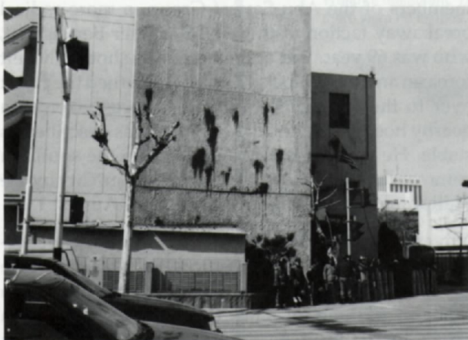
February 17, 1994—Taegu, South Korea: Views of the front entrance and side wall of the U.S. Consulate. Note the paint on the walls.
