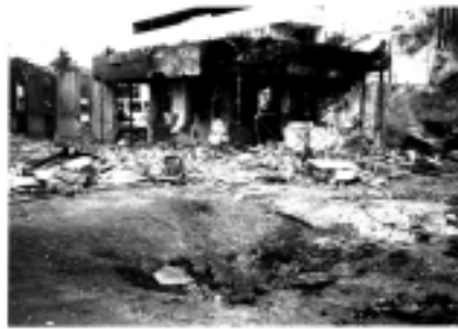
The blast crater and remains of the front gate house.
