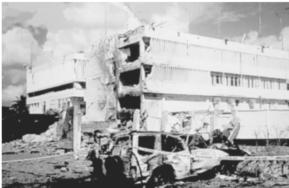
Damage to the U.S. Embassy in Dar es Salaam after the explosion.
