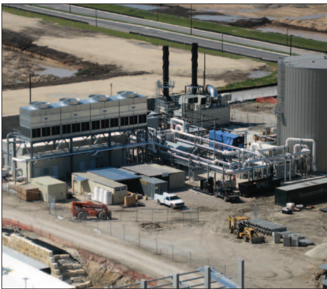
Combined Heat and Power: The new system provides the Dell's Children Hospital 100 percent of the thermal requirements to operate the hospital's power supply; and cleaner, more reliable power that has a power backup to the electric grid.
