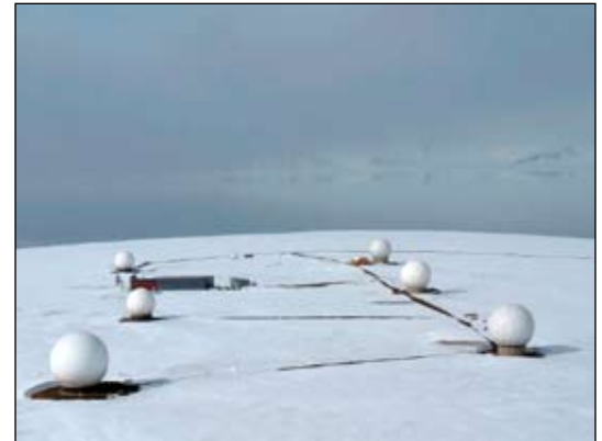
This picture is an aerial view of the operations building and the six protective radomes over the telemetry and command antennae at SvalSat. (Credit: KSAT)
