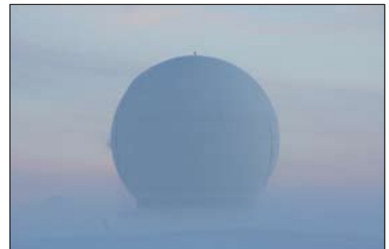
This picture shows typical conditions of early or late winter during which there is still daylight. The dome has ropes hanging from it to knock off accumulated snow. The tracking facility is on a plateau several hundred feet above the village of Longyearbyen. A snowcat plows the steeply switchbacked access road daily in winter; even so, the site may become isolated from town for days at a time due to avalanches across the road or severe storm conditions. (Credit: KSAT)
