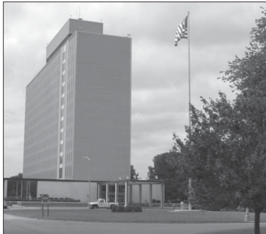
NIST’s 11-story Administration Building.
