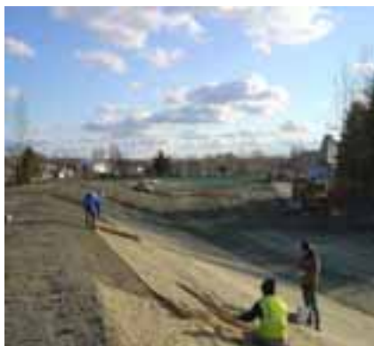
Laborers installing erosion control matting at the New Hampshire Plating site.
