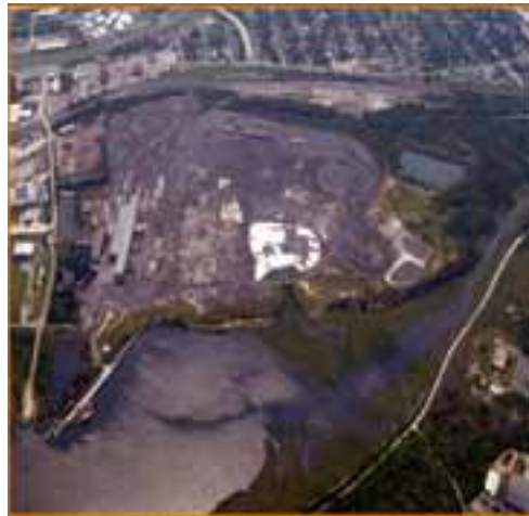
Aerial view of the Macalloy site after completion of all construction activities.
