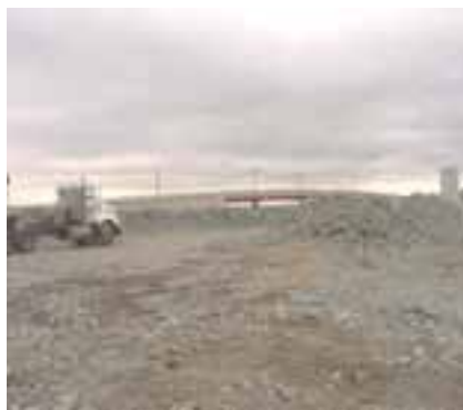
Truck atop Shattuck monolith prior to demolition.
