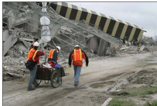
Division staff members map signals from transmitters buried in a collapsed building.
