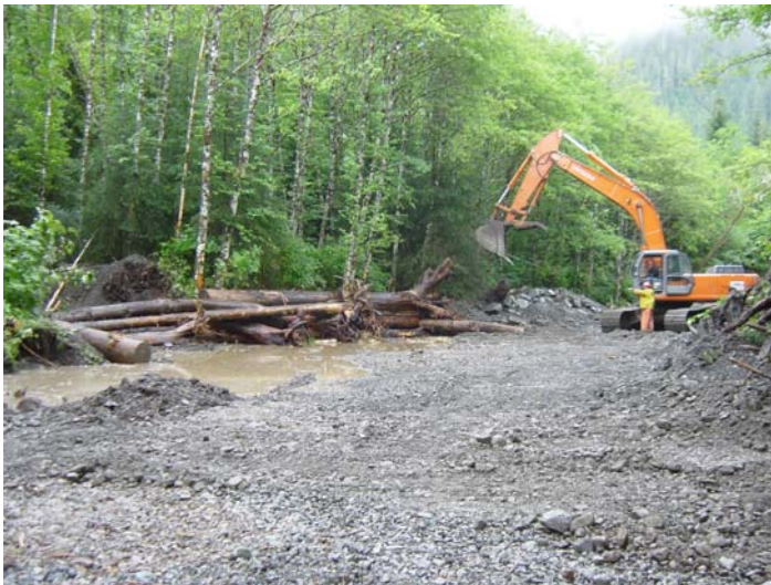
Photo 2. Photo of heavy equipment in-stream and mobilization of wood and rock occurring upstream of the bridge
